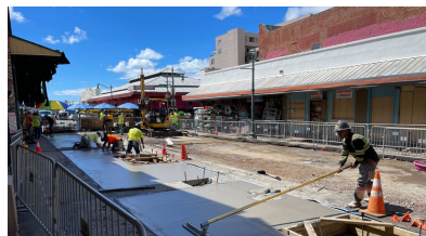
Above: Laying the cement for the future walkway of the Mall.
